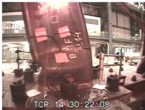
(c) 1 層中柱の局部座屈
