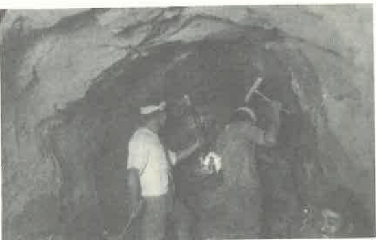
隧道掘削 (T. 11)
